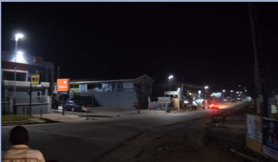
Street lights in Lokoja
