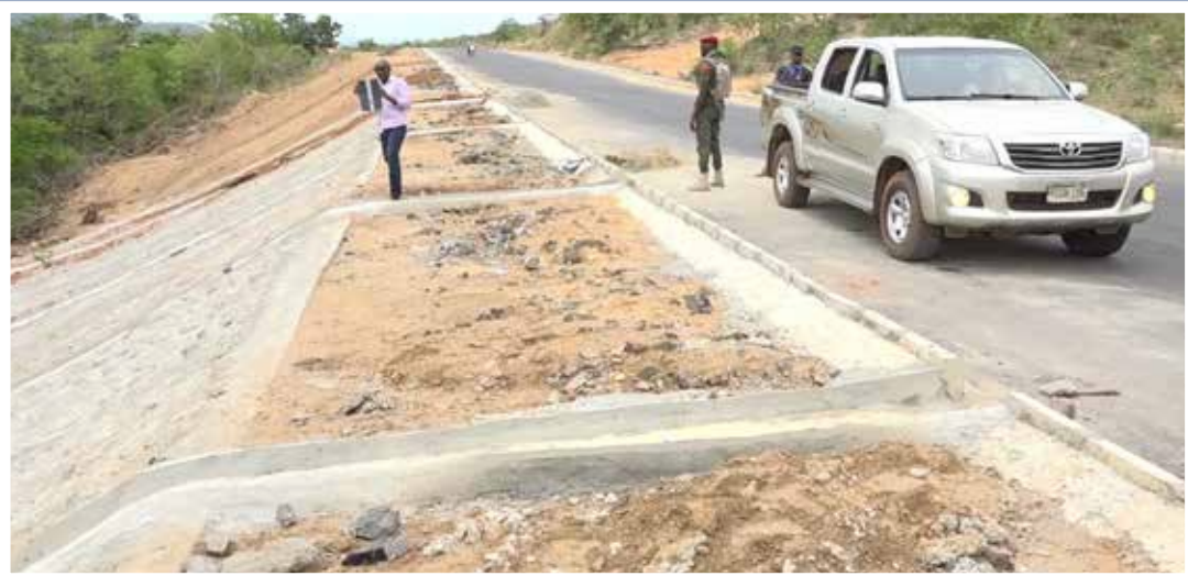
Umomi Erosion control
