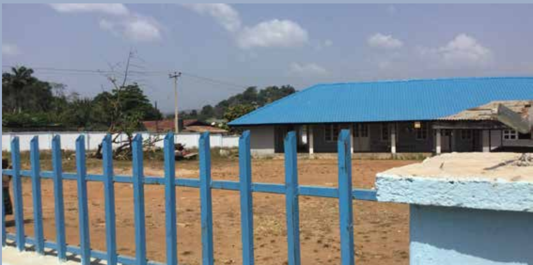
Renovation of PHC in Kabba, Kabba-Bunu LGA
