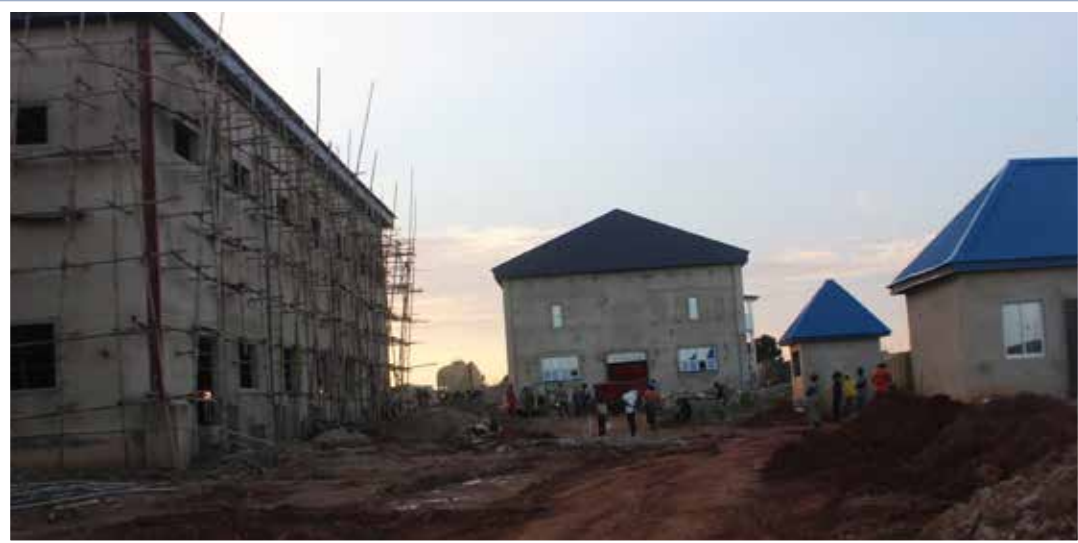
On-going construction at the Ejiba Rice Mill
