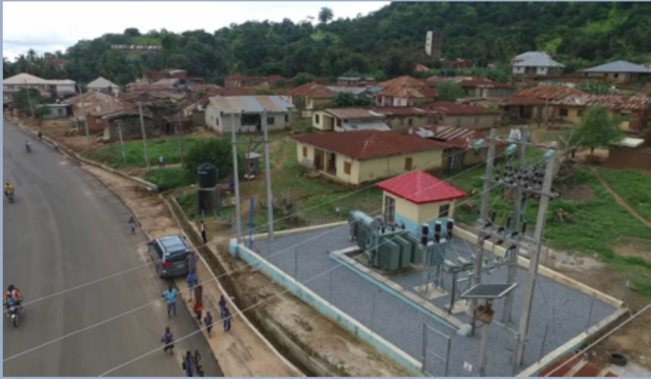
Ogori/Magongo power station
