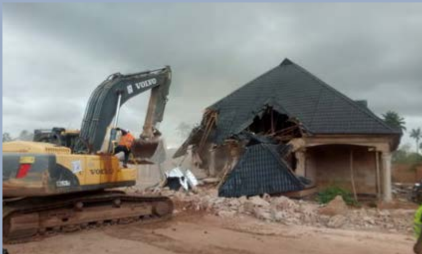
Demolition exercise of criminal houses/properties in Kogi State
