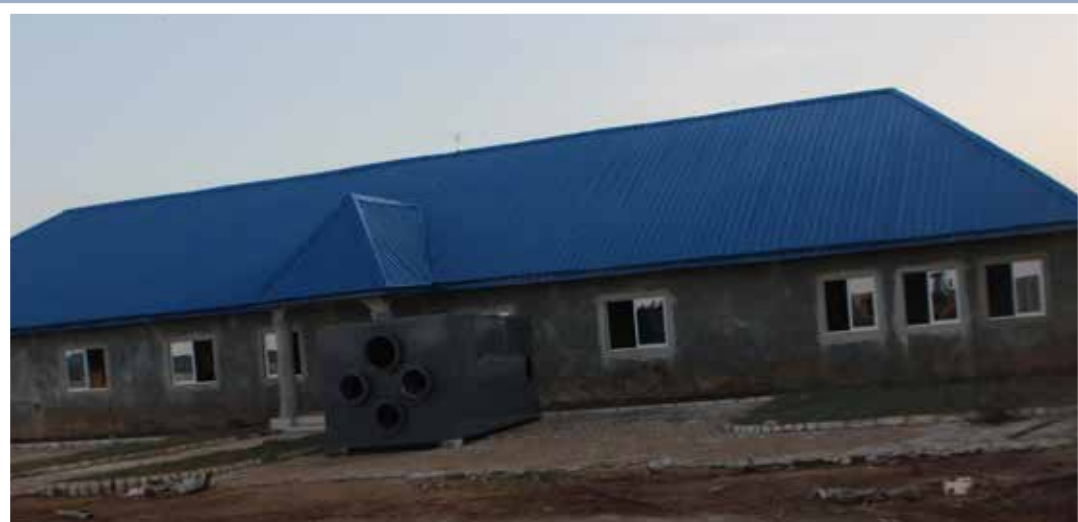
On-going construction at Ejiba Rice Mill in Kogi State
