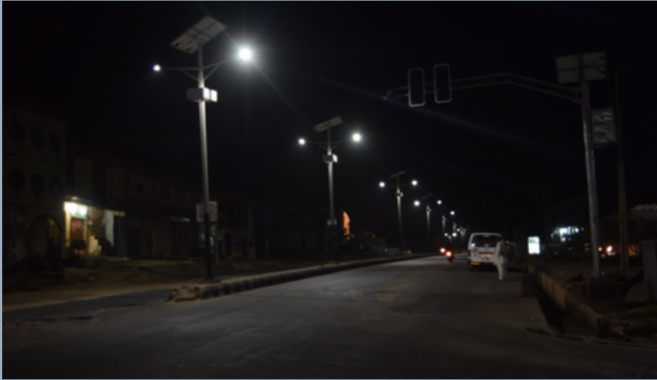
Installation of streetlight in Lokoja
