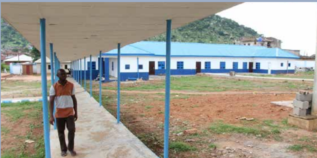
Renovated Okengwe General Hospital Complex in Okene LGA
