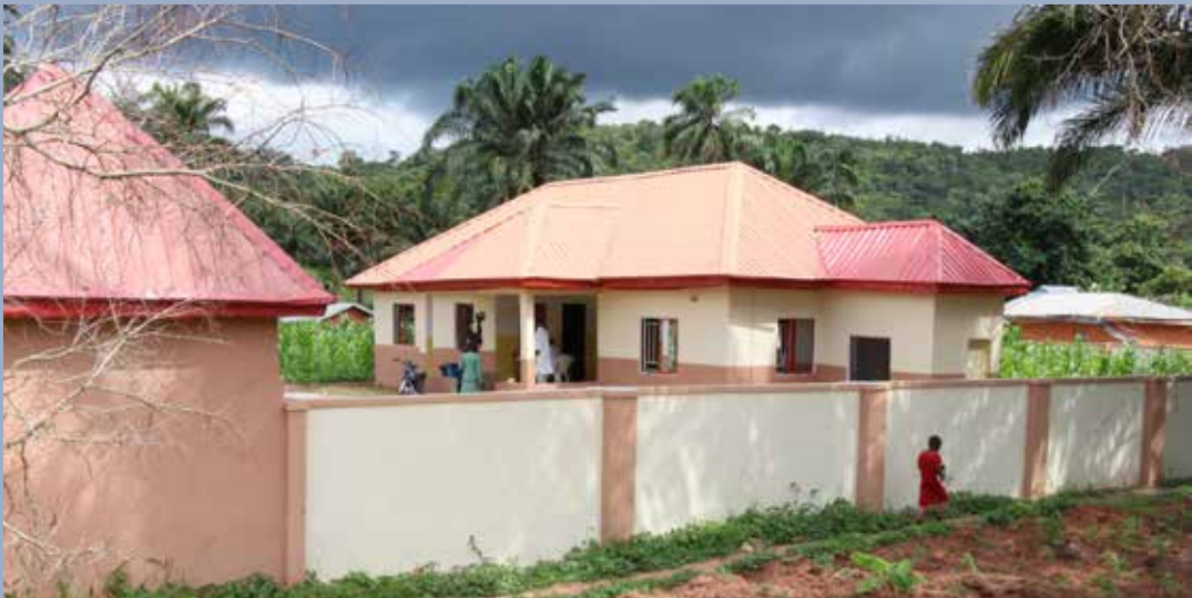
Newly constructed PHC, Emonyoku, Olamaboro LGA
