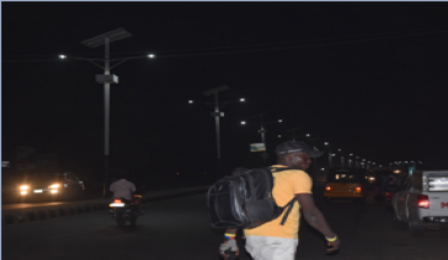
Newly installed Street lights in Lokoja
