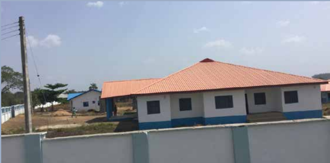
Renovation of PHC at Adogo, Ajaokuta LGA
