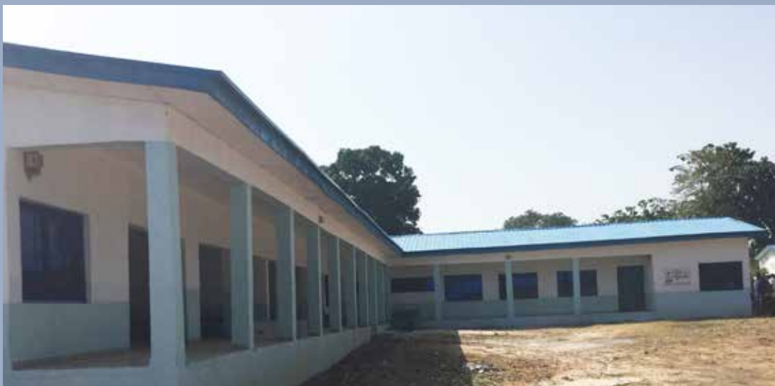
Part of the renovated Cottage Hospital in Gboloko, Bassa LGA
