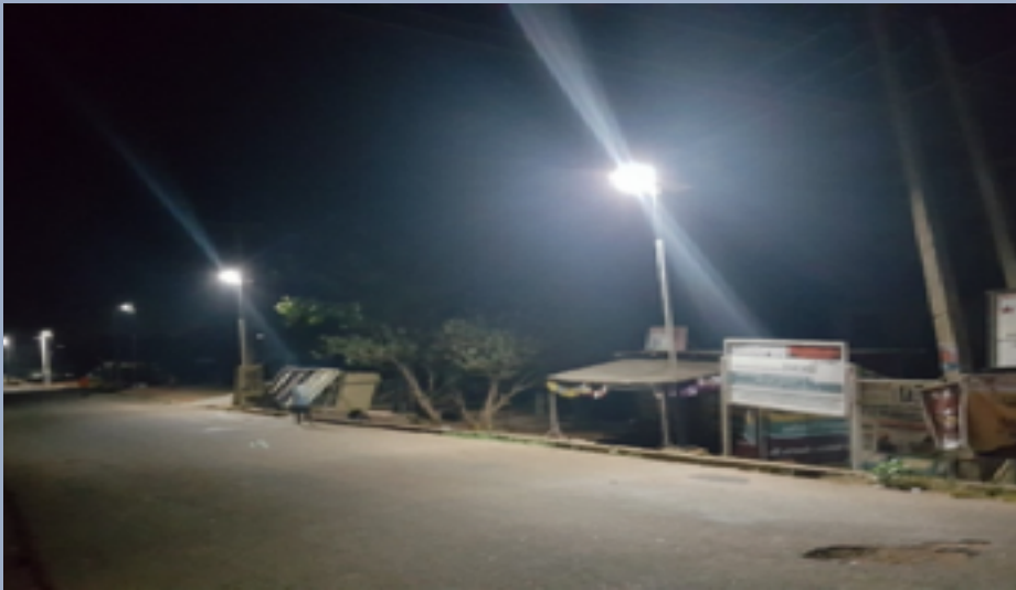
Street Light Installation in Lokoja Township
